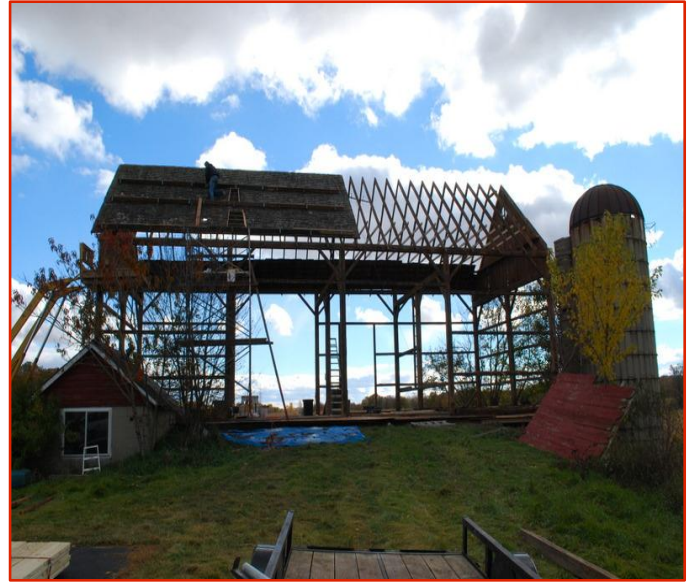
Barn being disassembled
