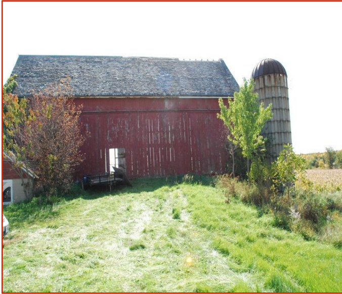
The Wendt Barn before disassembly
